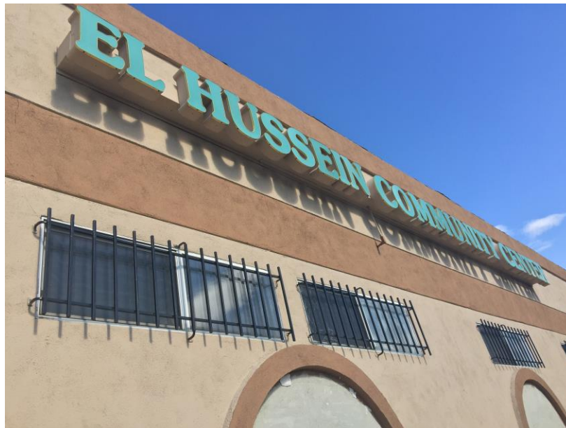
Figure 4. El Hussein Community Center. Located at 6840 Gage Avenue in Bell, the center served as BASTA’s primary meeting location. (Photo: Michael A. Moodian)
